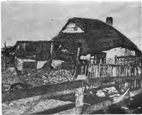
FIG. 23.—Enlarging the old house by adding part of a "bay," and extending the roof over it. A house at Burscough, England.
